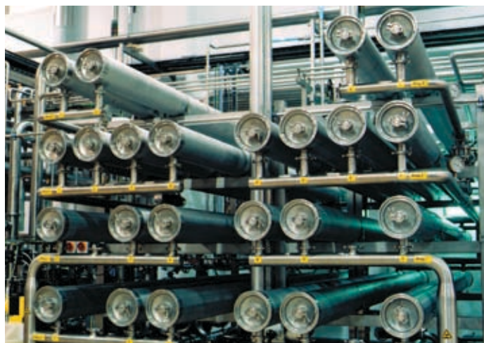
Figure 6: Membrane treatment plant recovering evaporative condensate for reuse (courtesy United Milk, now Westbury Dairies)
