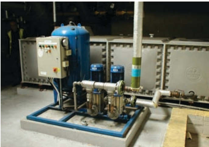
Figure 2: Typical booster pump unit (courtesy of Lyreco)
