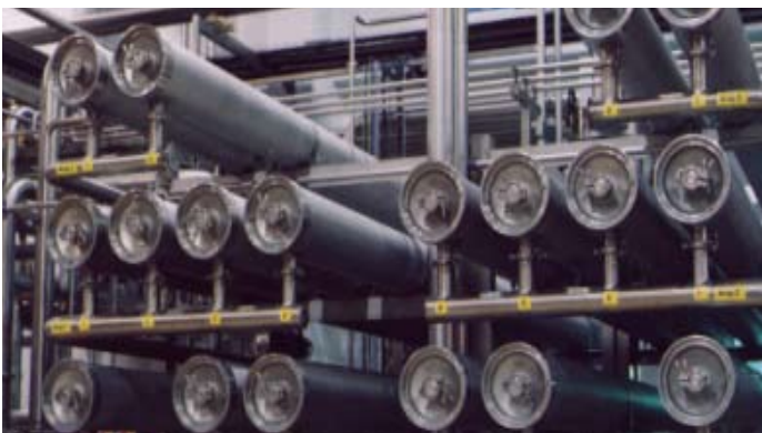
Figure 3: Membrane treatment plant recovering evaporative condensate for reuse (courtesy United Milk, now Westbury Dairies)
