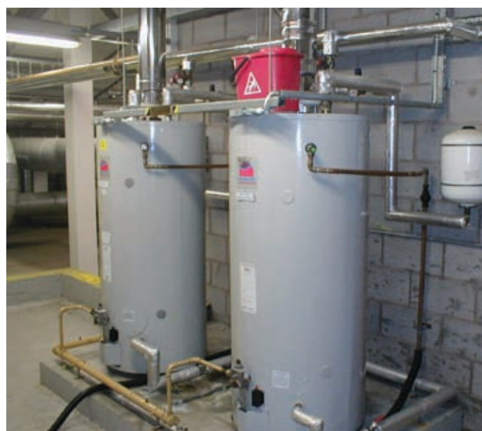
Figure 1: Typical self-contained gas-fired storage water heaters (courtesy of Lyreco)
