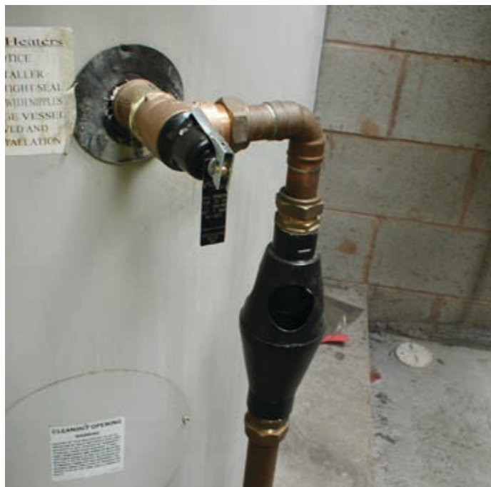
Figure 3: Relief valve and tundish on hot water heater (courtesy of Lyreco)
