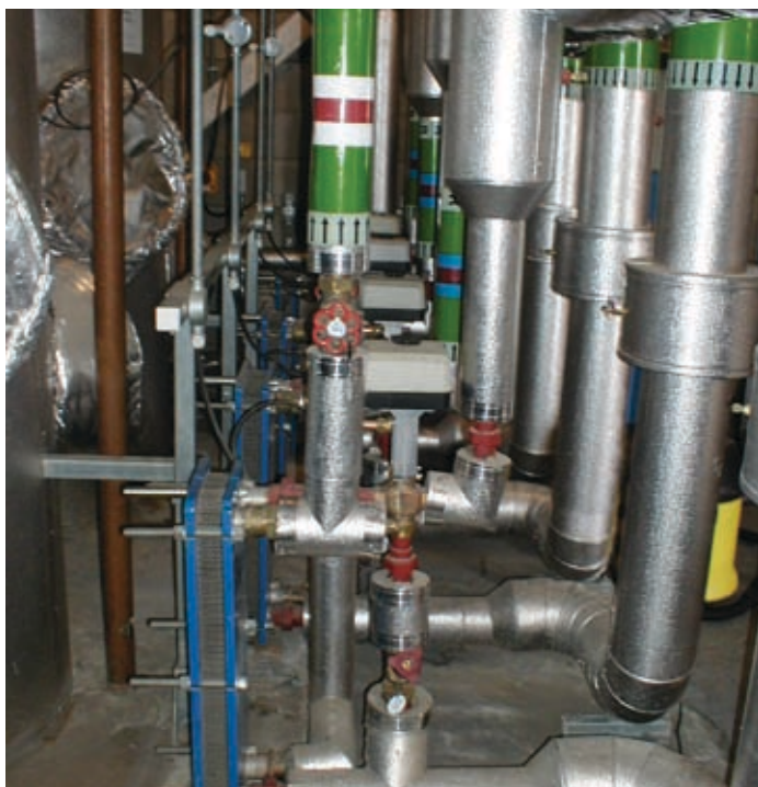
Figure 2: External plate heat exchangers (courtesy of Radisson)
