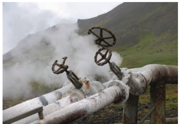
Figure 4: Steam leaks from faulty valves on unlagged steam lines
